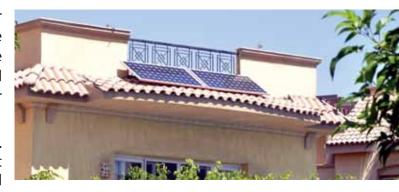
than PV modules power, smart inverters compensate the difference from the grid, otherwise, excess power from PV modules goes directly to batteries for recharging. In the occasion of grid power cutoff during daytime, PV modules electricity goes directly to home local grid to operate home appliances, however, if home load is larger than PV modules power, the difference is compensated from the charged batteries, otherwise, the excess from PV modules goes directly to batteries for recharging.
